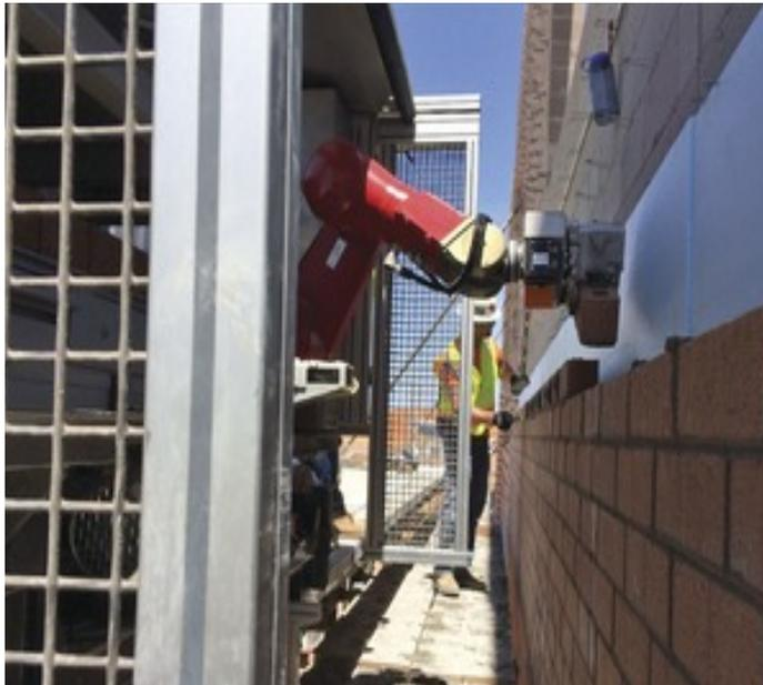
A robot that lays bricks is now out of beta testing and at work alongside masons and laborers at a school-building jobsite in Ft. Collins, Colo. The Semi-Autonomous Mason, more commonly known as SAM, is already booked for two
